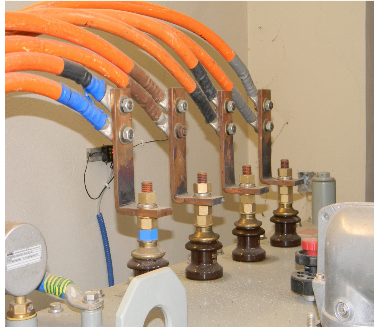
High- low tension connection Same GSHT-system as Sogakope
